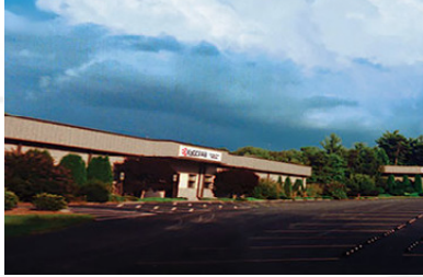
North Carolina Facility (USA)
