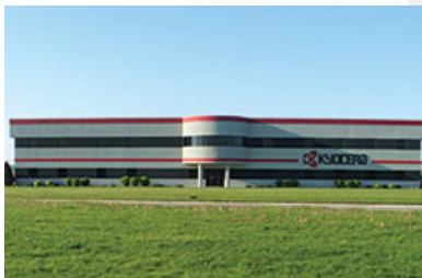
Ohio Facility (USA)
