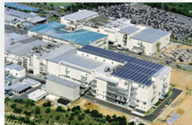
Yokaichi Facility (JAPAN)
