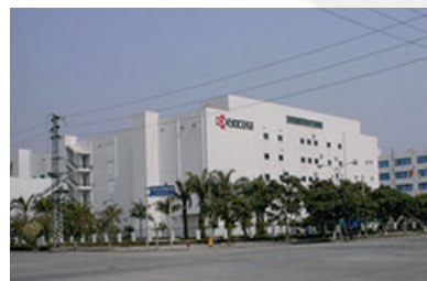
Silong Facility (CHINA)
