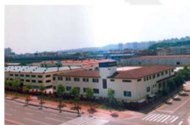
Incheon Facility (KOREA)
